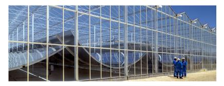
1GW solar thermal system for Enhanced Oil Recovery in Oman
